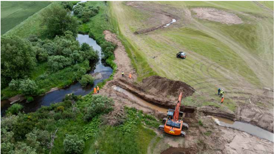
Restoration work gets underway on the River Breamish
