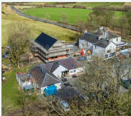
Construction underway on the Crook Inn Bunkhouse at Tweedsmuir
