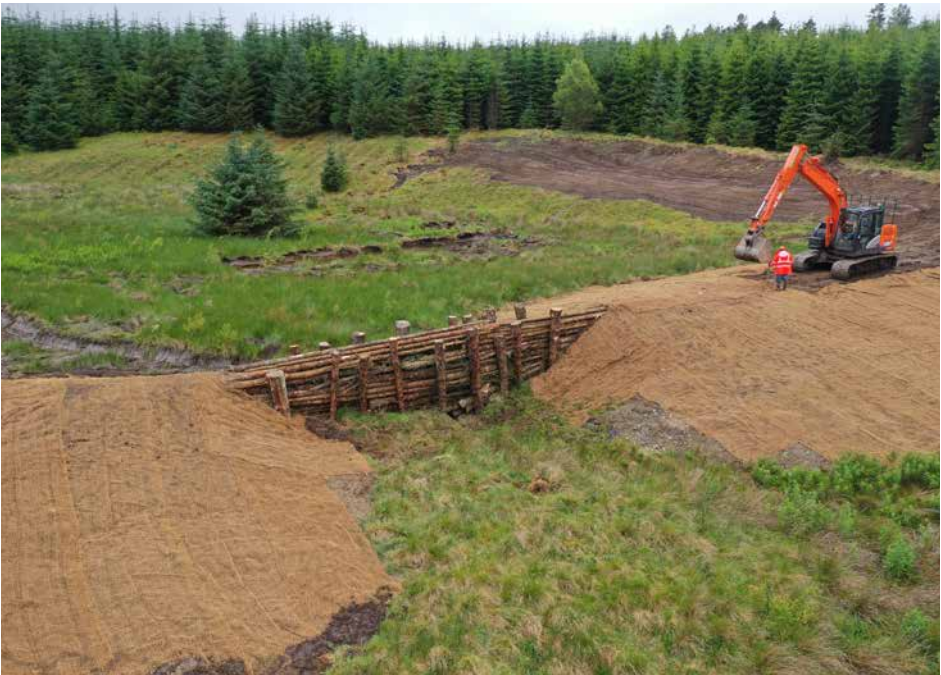
Installation of the flood attenuation bund on the Middle Burn
