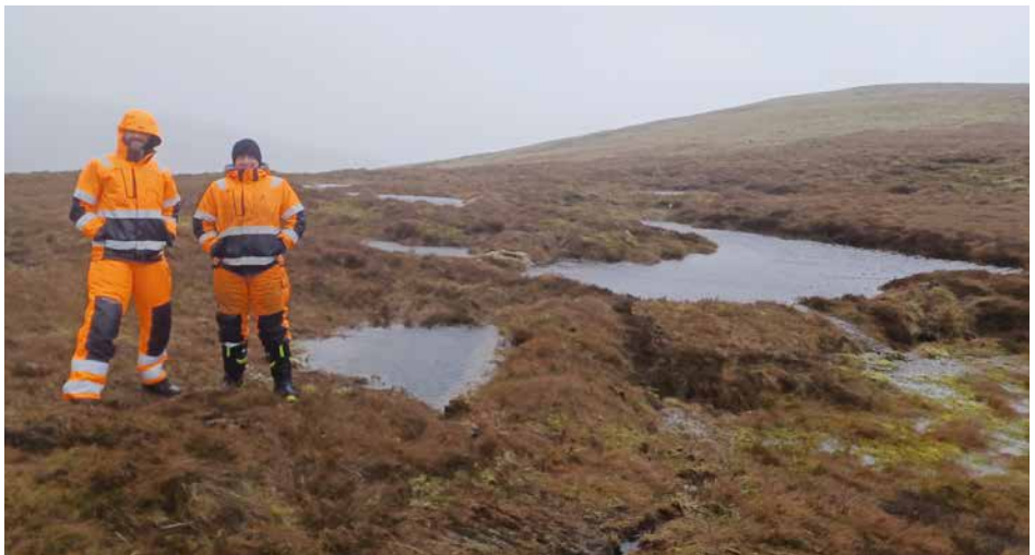
This winter, specialist contractors undertook hag reprofiling and peat bunding works at Wemyss & March Estate; the bunding work (pictured) will slow the flow of water through the peatland and create important bog pool habitat which will benefit a variety of wildlife
