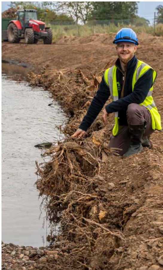
Craig Marshall (Senior Project Officer, Tweed Forum) is pictured during the installation of timber root-wads, a more sustainable solution to stabilising riverbank erosion on the Wooler Water
