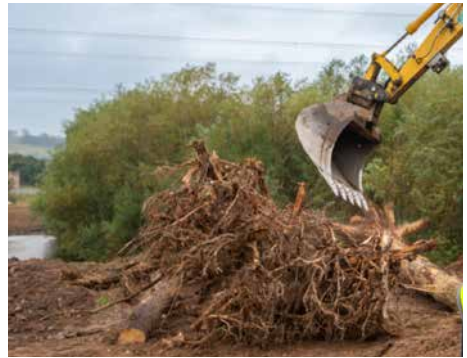
Installation of timber root-wads
