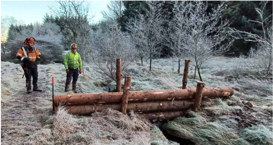
One of the newly installed log jams on the Middle Burn, a tributary of the Eddleston Water
