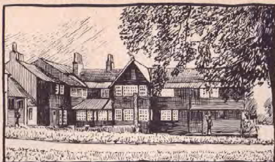
The attractive timber-faced front of Skirling House, on the village green.
